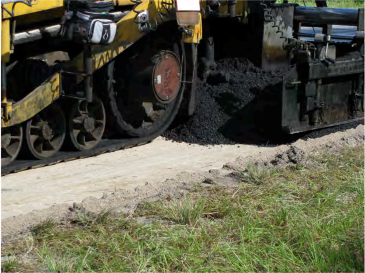
Spreading asphalt over a phosphogypsum road base.
