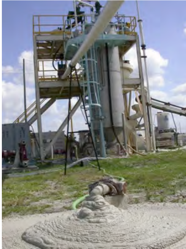
Deep cone pilot plant with thickened clay paste.
