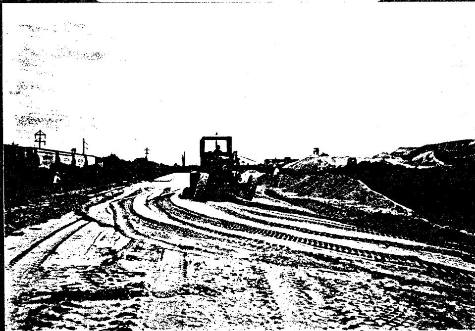
MOTOR GRADER BLADING ROAD
