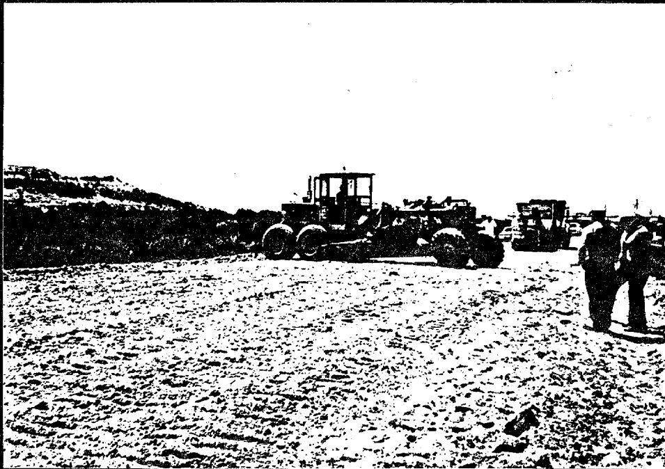
MOTOR GRADER BLADING ROAD
