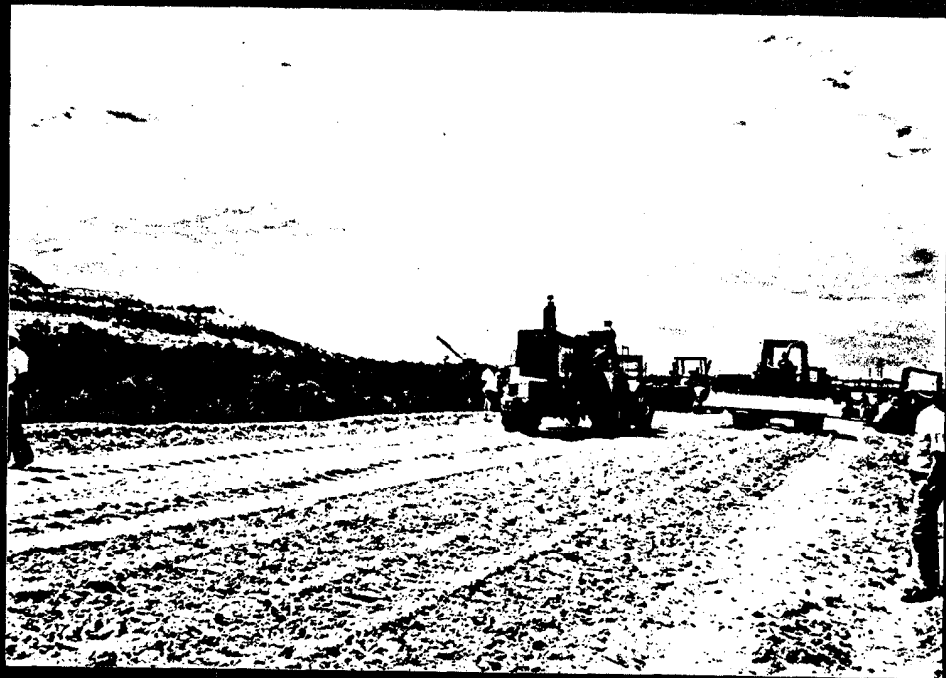
BULLDOZER PASSING OVER ROAD TO BREAK LUMPS IN GYPSUM
