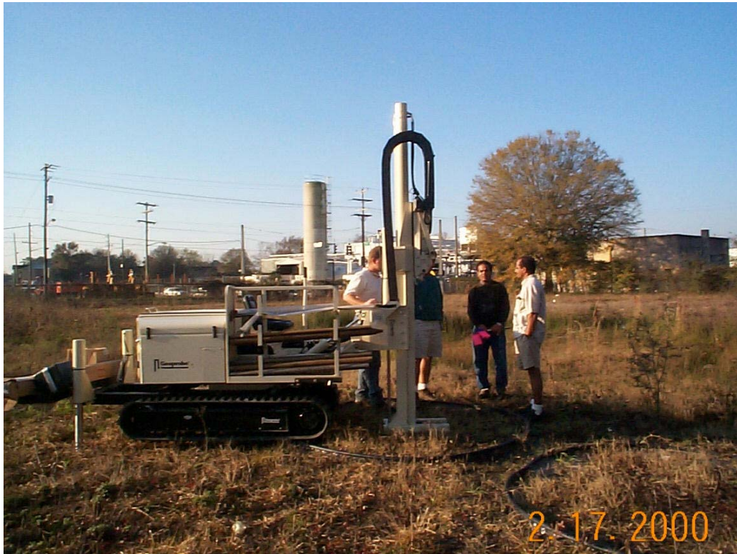
Figure 29. Geoprobe Used for Well Installation in the Jacksonville Demonstration Site.
