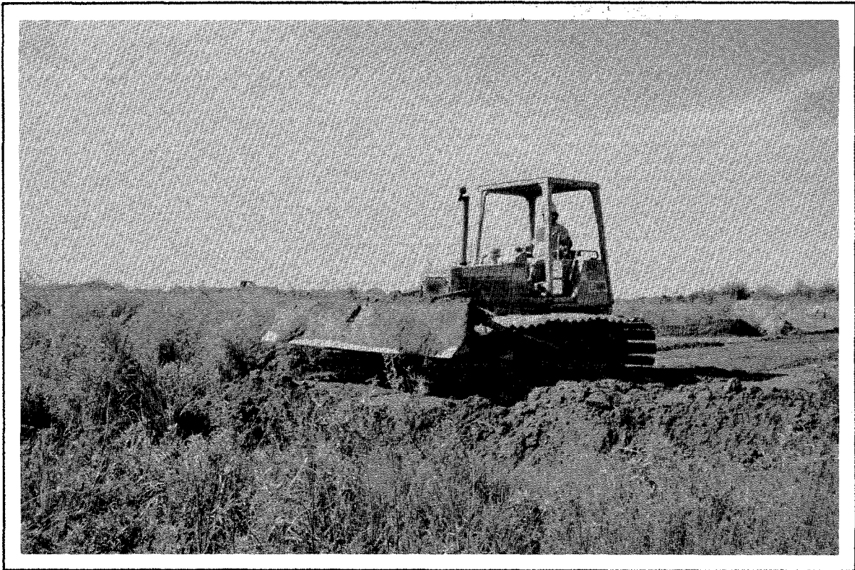
PLACEMENT OF FILL PAD
