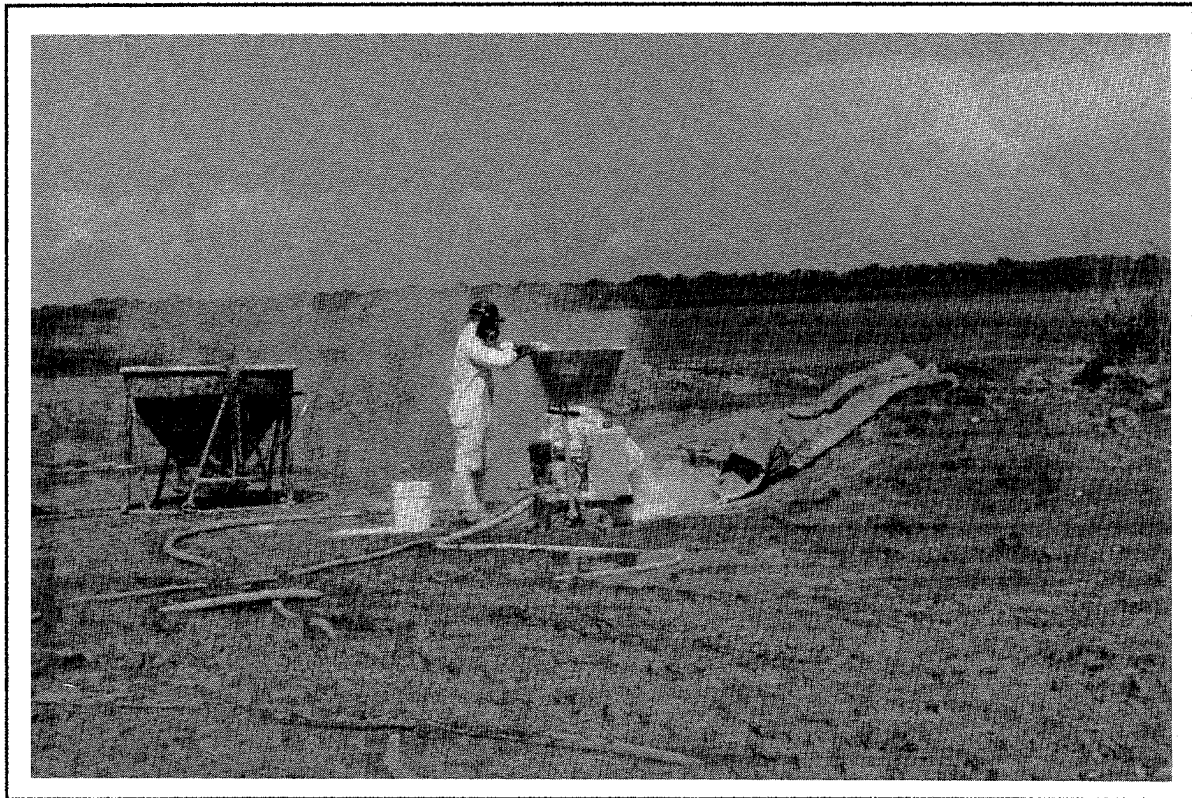
FIGURE 13 QUICKLIME PREPARATION AND INJECTION USING COMPRESSED AIR
