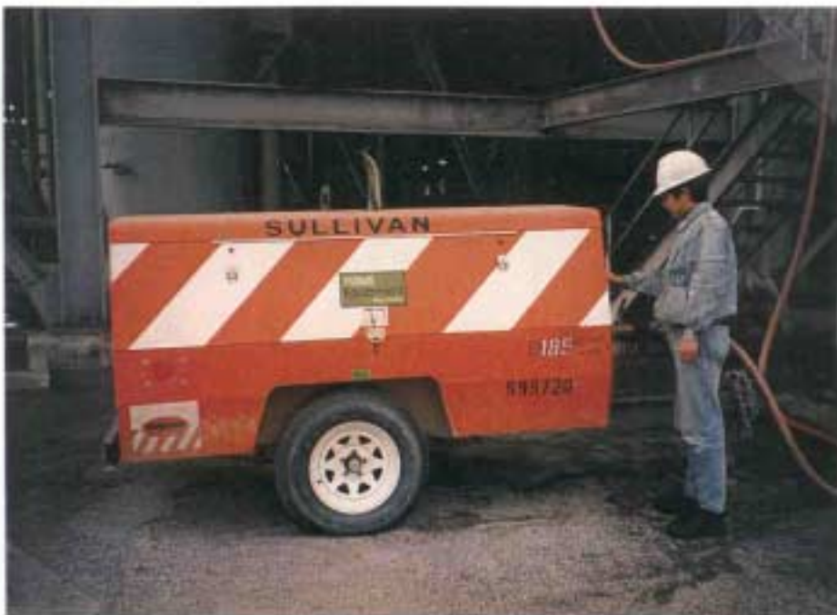
Figure 41. Air Compressor for 6-Inch ASH Air Supply.
