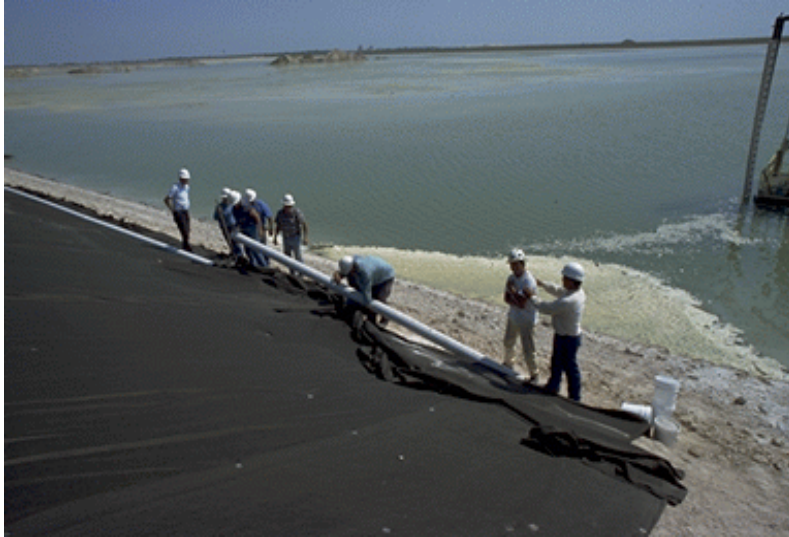
Figure 7(c). Installation of Toe Drain for Northern Geodrain Test Section. [04/14/99: 20]
