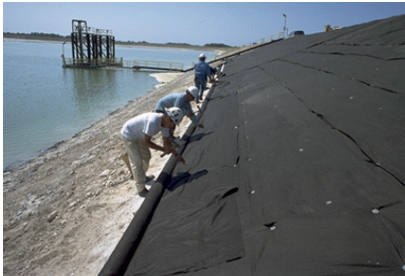
Figure 7(d). Installation of Toe Drain for Northern Geodrain Test Section. [04/14/99: 23]
