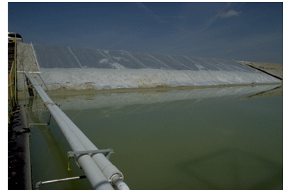
Figure 25(e). May 28, 1999; t = +32 days Pond Level = 127.7 ft msl [06/21/99: 13]
