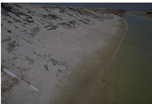
Figure 23(t). Mar 14, 2000; t = +323 days Pond Level = 135.6 ft msl [04/06/00: 19]
