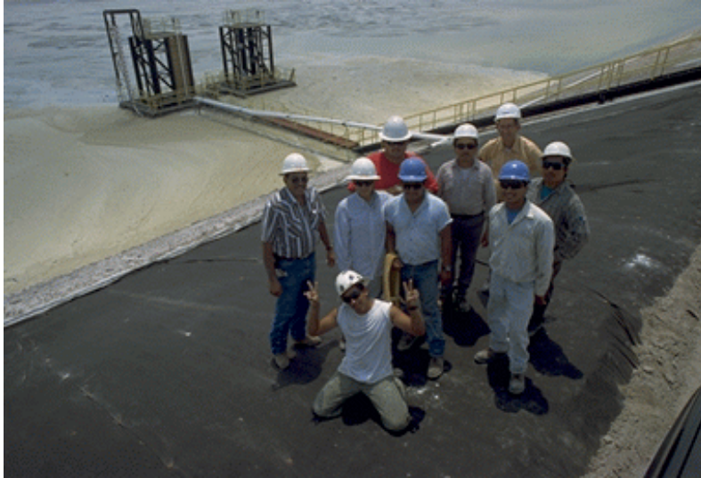
Figure 21(a). Geodrain Installation Completed. Apr 26, 1999; t = 0 days; Pond Level = 125.8 ft msl [06/08/99: 7]
