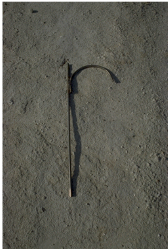
Figure 8. Closeup of Welded Anchor Used to Hold Toe Drains and Conveyance Pipeline from Southern Geodrain Test Section. Apr 18, 1999; t = -8 days; Pond Level = 125.4 ft msl [04/28/99: 25]
