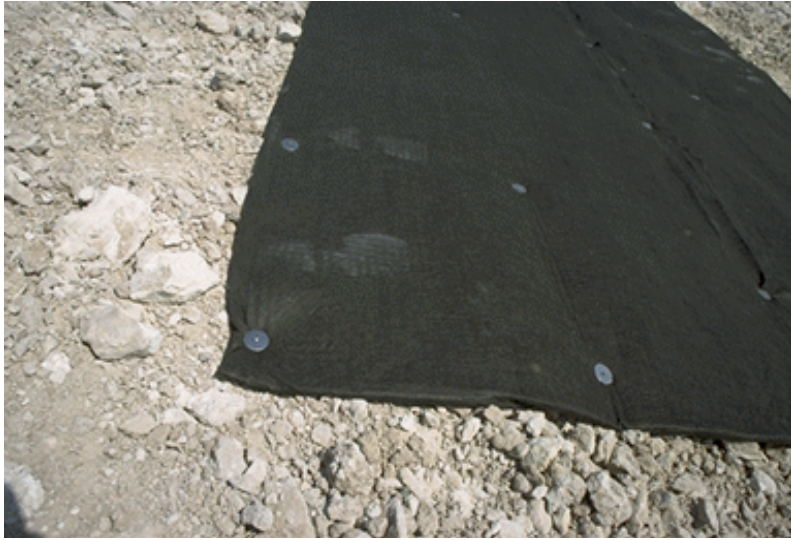
Figure 3. Nailing Geodrain to Embankment. Apr 05, 1999; t = -21 days; Pond Level = 124.1 ft msl [04/12/99: 35]
