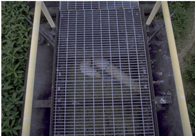
Figure 20. Repaired Elbows under Catwalk. May 29, 2001; t = +773 days; Pond Level = 135.8 ft msl [07/20/01: 5]
