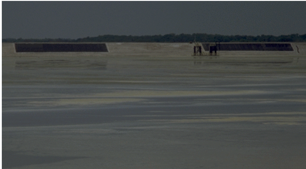
Figure 21(b). Geodrain Installation Viewed from East Embankment. Apr 26, 1999; t = 0 days; Pond Level = 125.8 ft msl [06/08/99: 18 (enlargement)]
