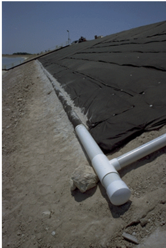
Figure 11(b). Standpipe N-1 at North End of Northern Geodrain Test Section. [04/14/99: 28]
