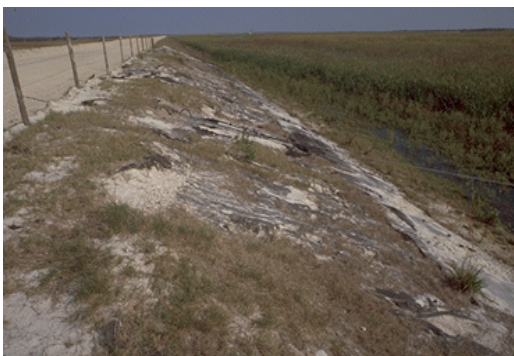
Figure 22(aa). Feb 22, 2001; t = +668 days Pond Level = 136.9 ft msl [03/14/01: 32]
