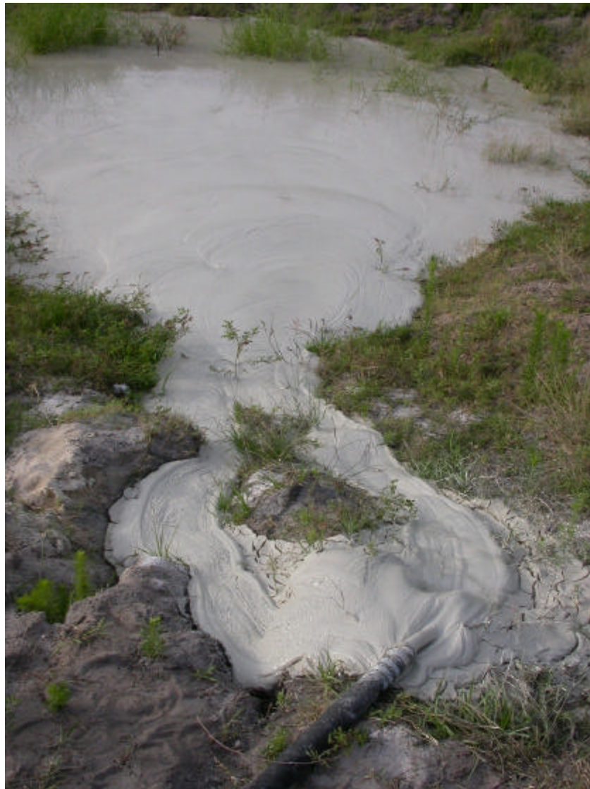
Figure 96. Paste Storage Pond Near the End of Field Testing Period.
