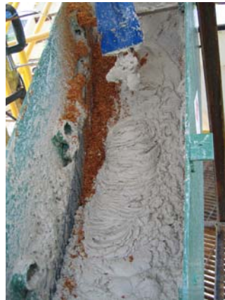
Dewatered Sand/Clay Mix on the Static Screen
