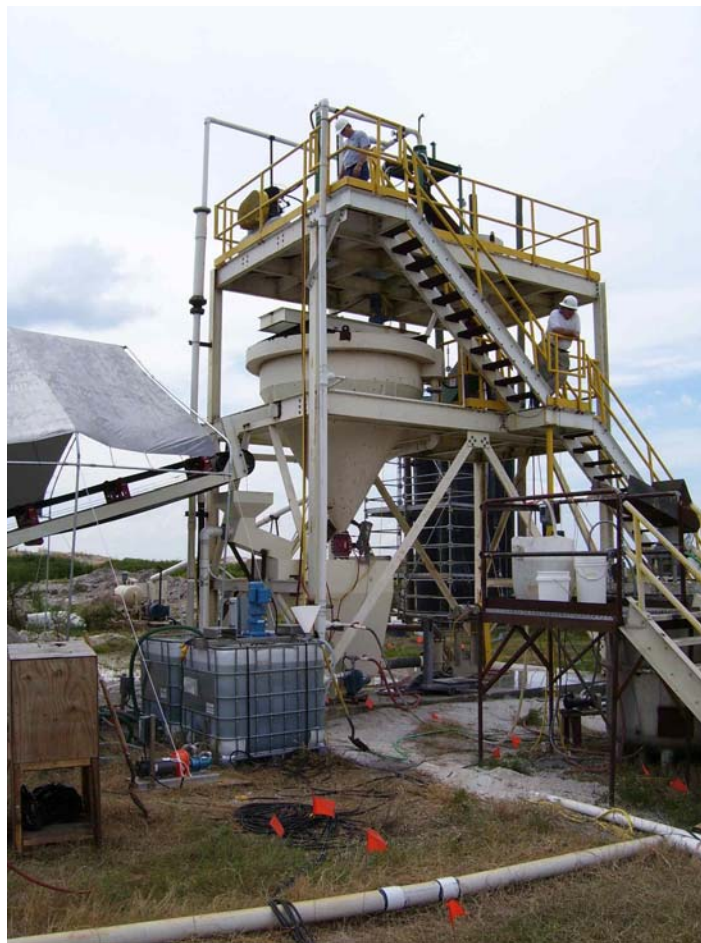
Figure 12. Upgrading of the Pre-Existing FIPR/DIPR Sand/Clay Mix and Dewatering Pilot Plant.
