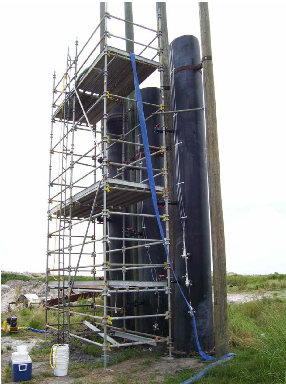
Figure 14. Scaffolding to Provide Access for Measurements of Water and Clay Levels.
