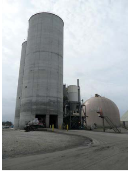
Figure 9. TECO “Big Bend” Power Plant.
