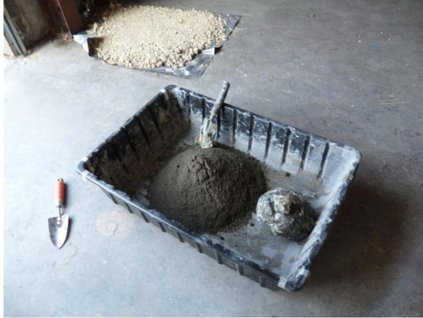
Figure 11. Mixing Materials in Mortar Box.
