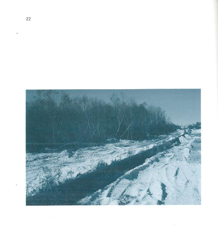
Figure 7. Initiation of capping of 9-year-old clay settling pond with sand tailings, Florida. Trees being crushed and covered (upper left) are the results of natural succession over the 9 year interval.
