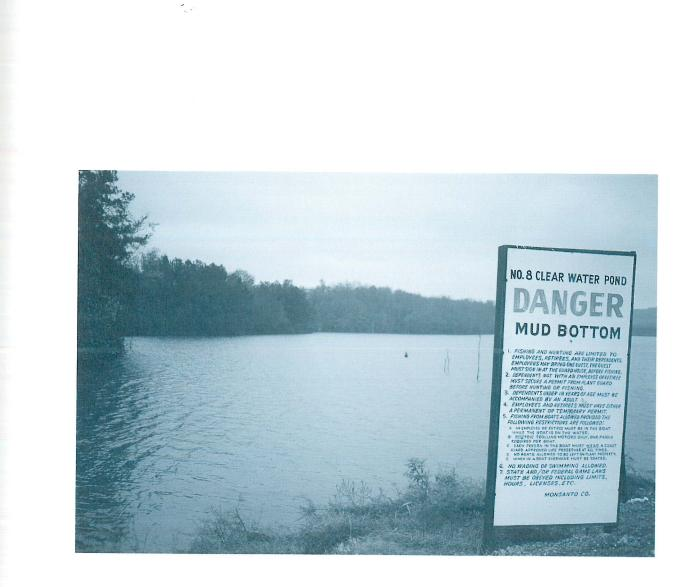
Figure 29. A deep slurry pond used to clarify water used in phosphate processing in Tennessee.
