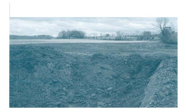
Figure 13. Tennessee phosphate mine recently filled and graded for planting soon after completion of mining.
