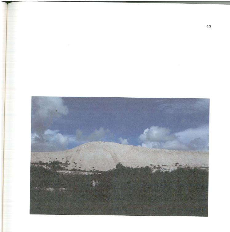
Figure 19. A typical stack of phosphogypsum, a by-product of fertilizer production, being stored on the landscape in Florida.
