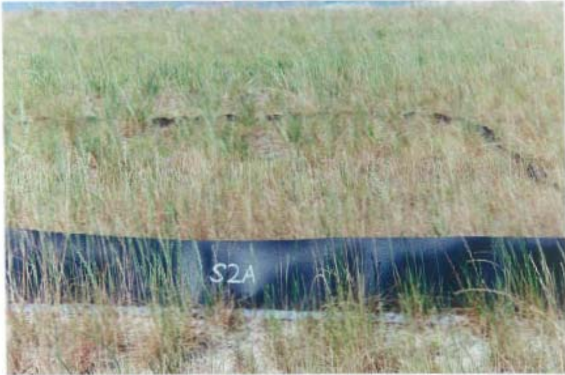
Photograph I-21. Side Slope Test Plot S2A on 04/27/99 (T=208 Days).
