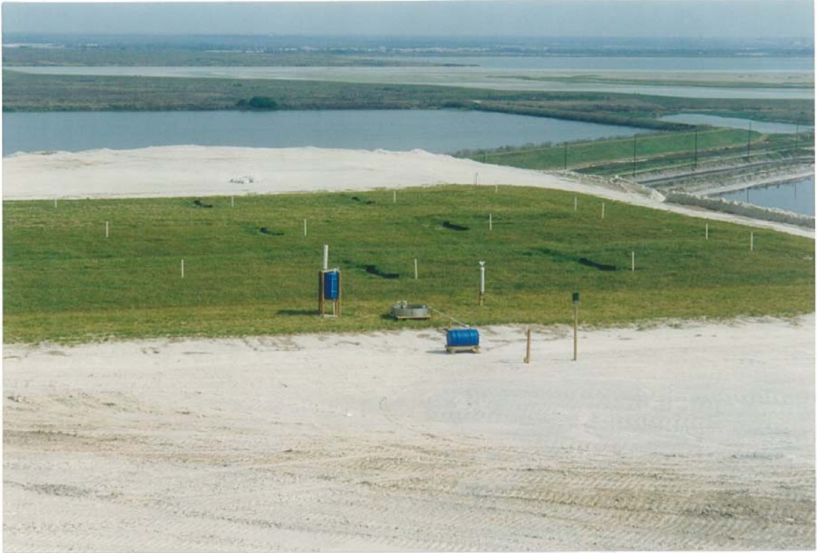
Photograph K-9. Top Gradient Test Plots on 02/10/99 (T = 131 Days).
