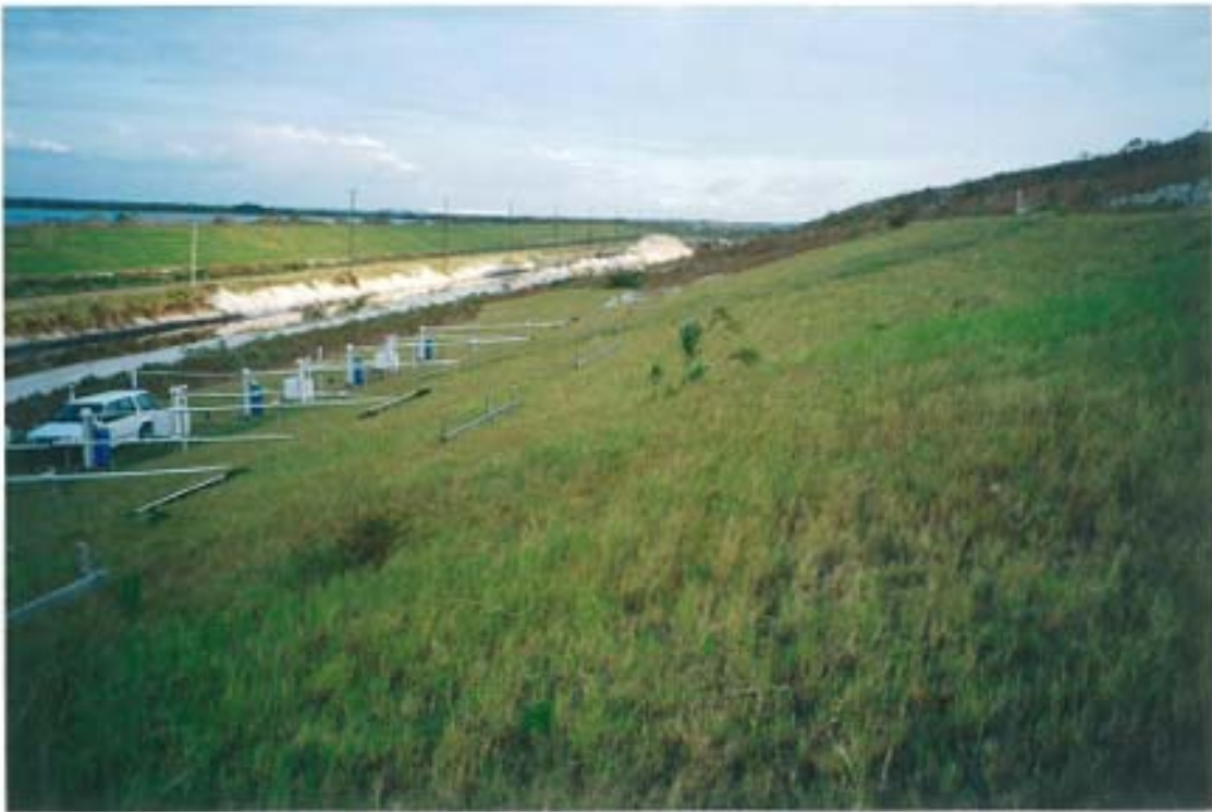
Photograph I-50. Side Slope Test Plots on 11/14/01 (T=1140 Days).
