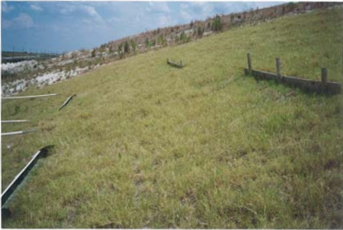
Photograph I-43. Side Slope Test Plot S1A on 06/01/01 (T=974 Days).
