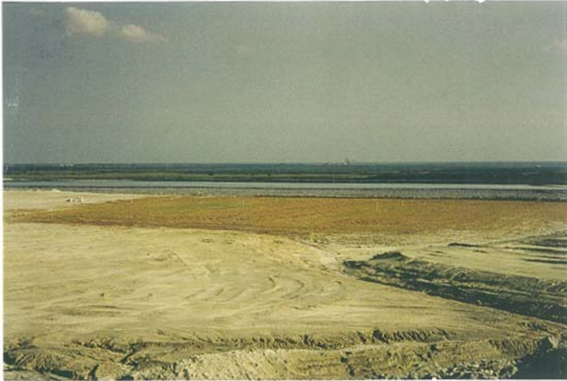
Photograph K-1. Top Gradient Test Plots on 10/15/98 (T = 14 Days).
