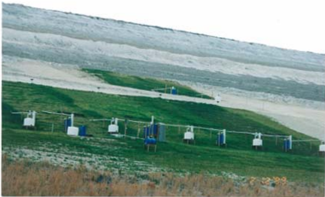
Photograph I-12. Side Slope Test Plots on 02/10/99 (T=132 Days).
