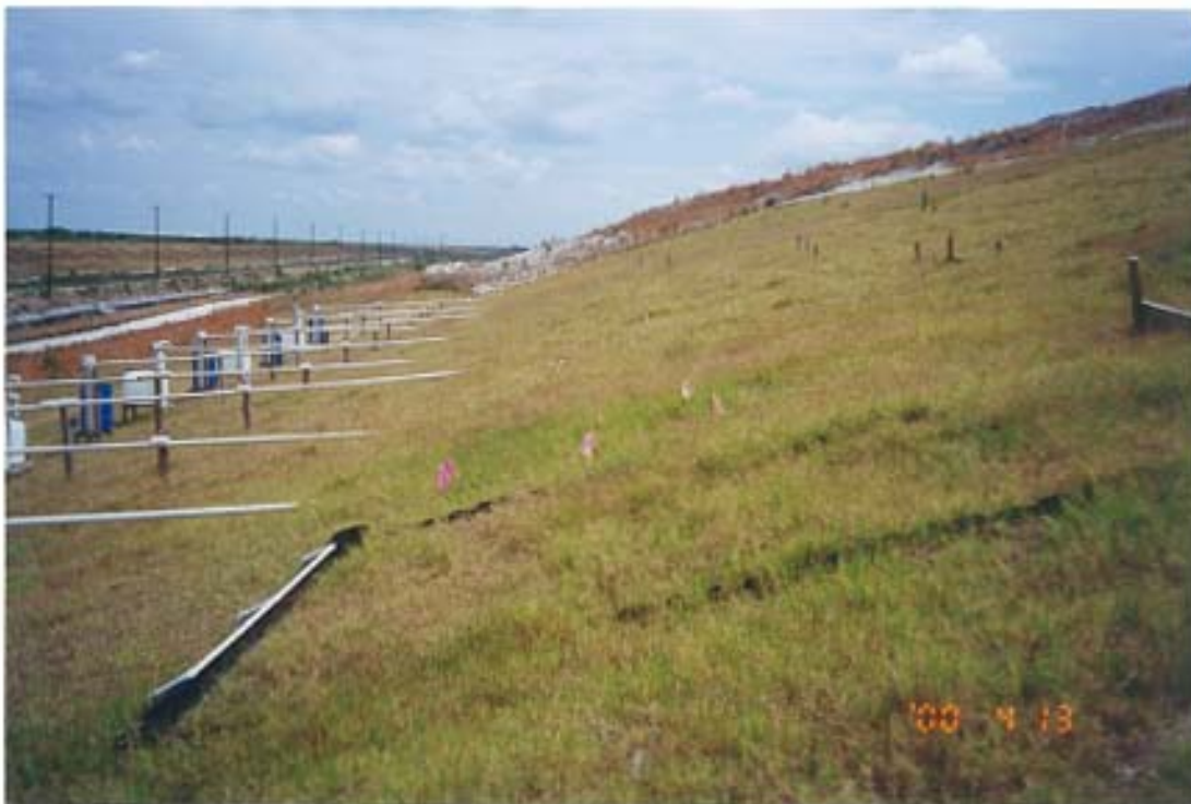
Photograph I-31. Side Slope Test Plots on 04/13/00 (T=560 Days).
