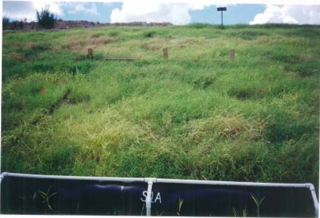
Photograph I-25. Side Slope Test Plot S1A on 09/09/99 (T=343 Days).
