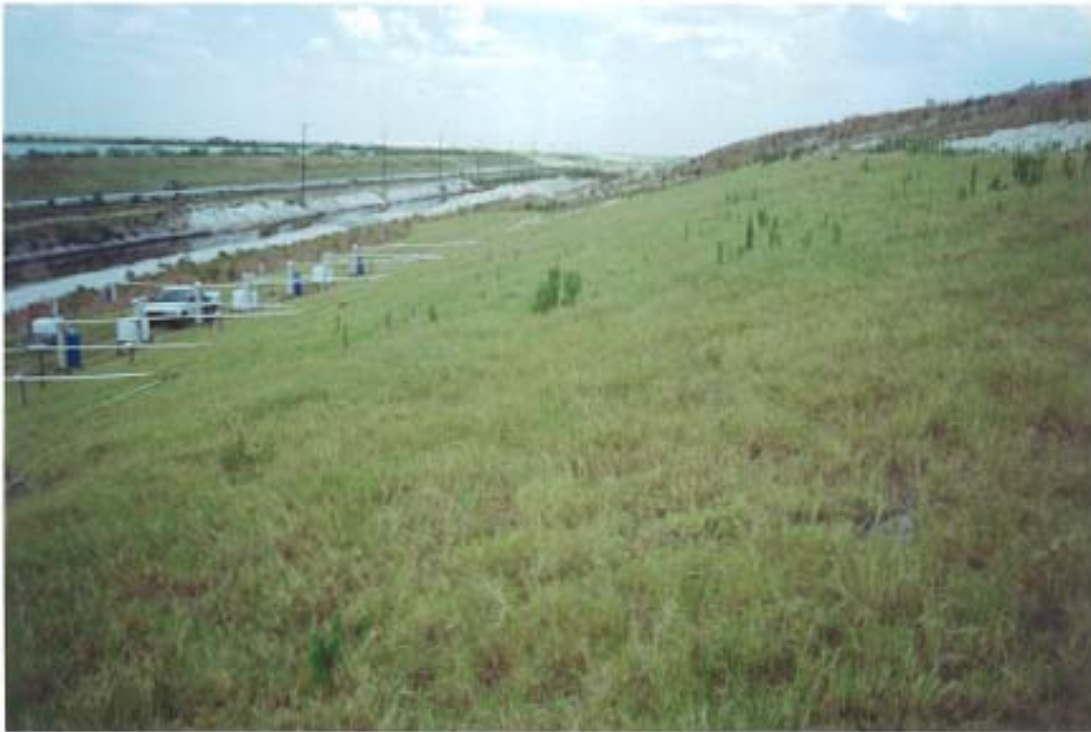
Photograph I-42. Side Slope Test Plots on 06/01/01 (T=974 Days).
