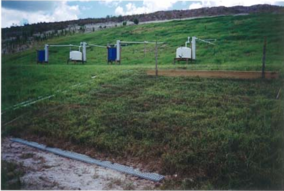
Photograph I-23. Additional Side Slope Runoff Collector S3A Installed July 1999.
