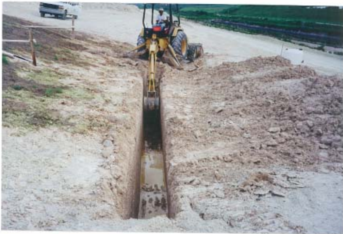
Photograph I-22. Excavating Toe Ditch at Side Slope Test Plot S2C on 07/01/99.
