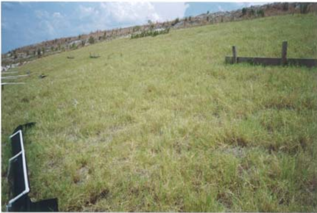
Photograph I-44. Side Slope Test Plot S2A on 06/01/01 (T=974 Days).
