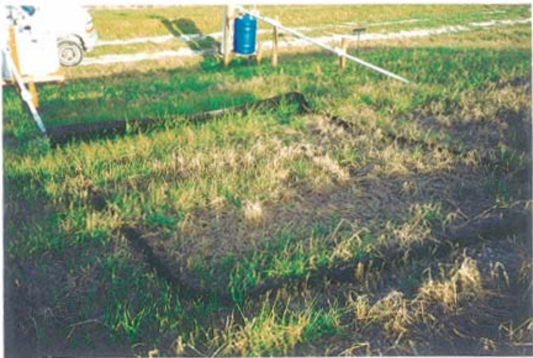
Photograph I-6. Side Slope Test Plot S2A on 01/13/99 (T=104 Days).
