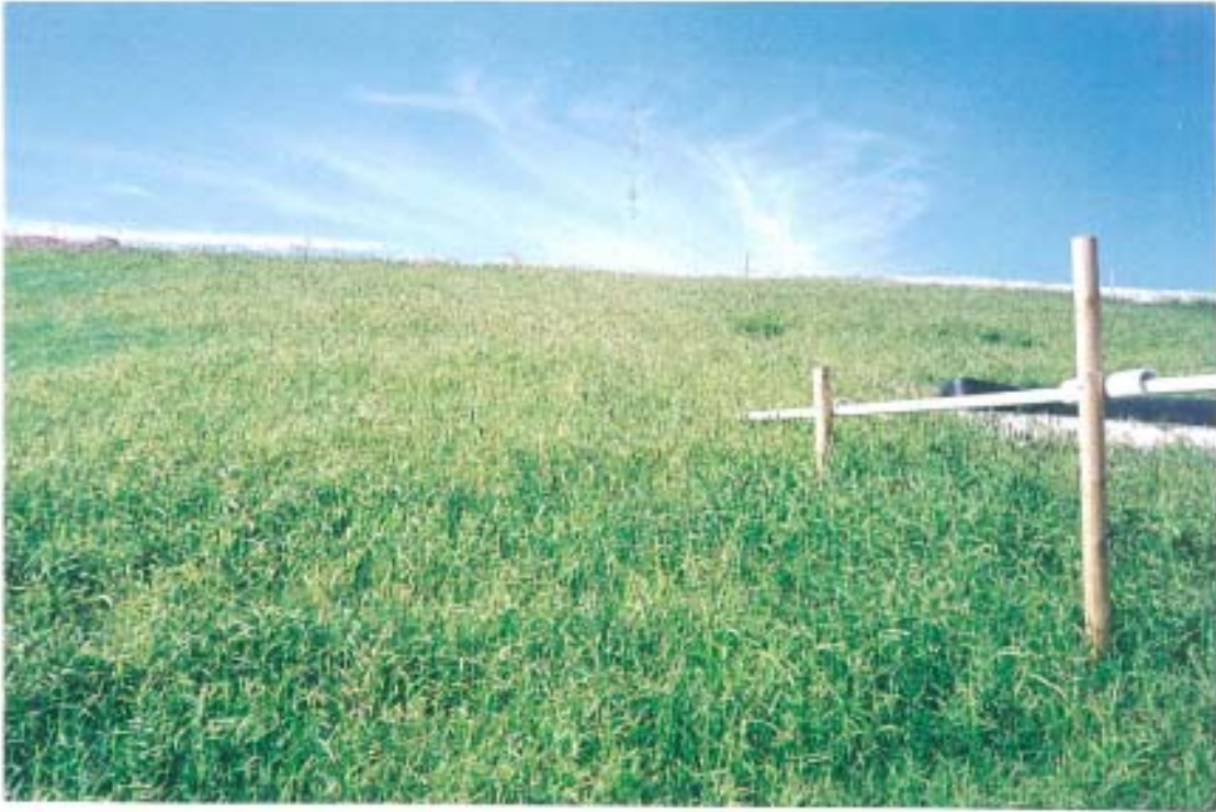
Photograph I-1. Side Slope Test Plot S2A on 11/12/98 (T=49 Days).
