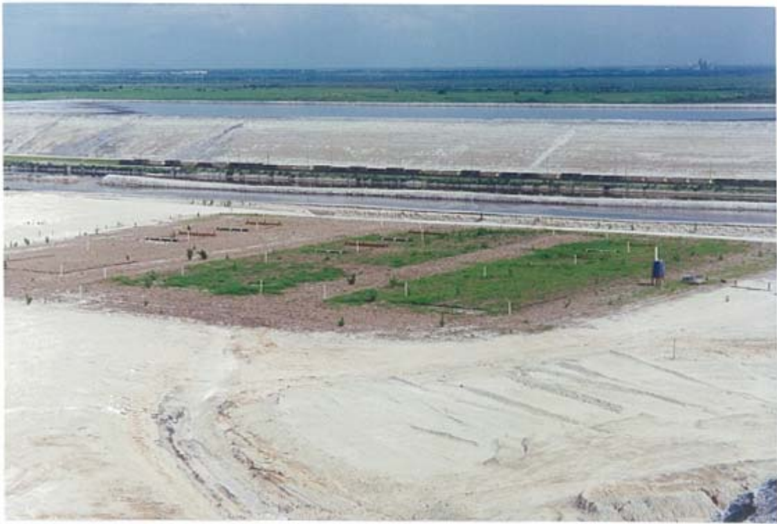
Photograph K-13. Top Gradient Test Plots on 07/01/99 (T = 272 Days).
