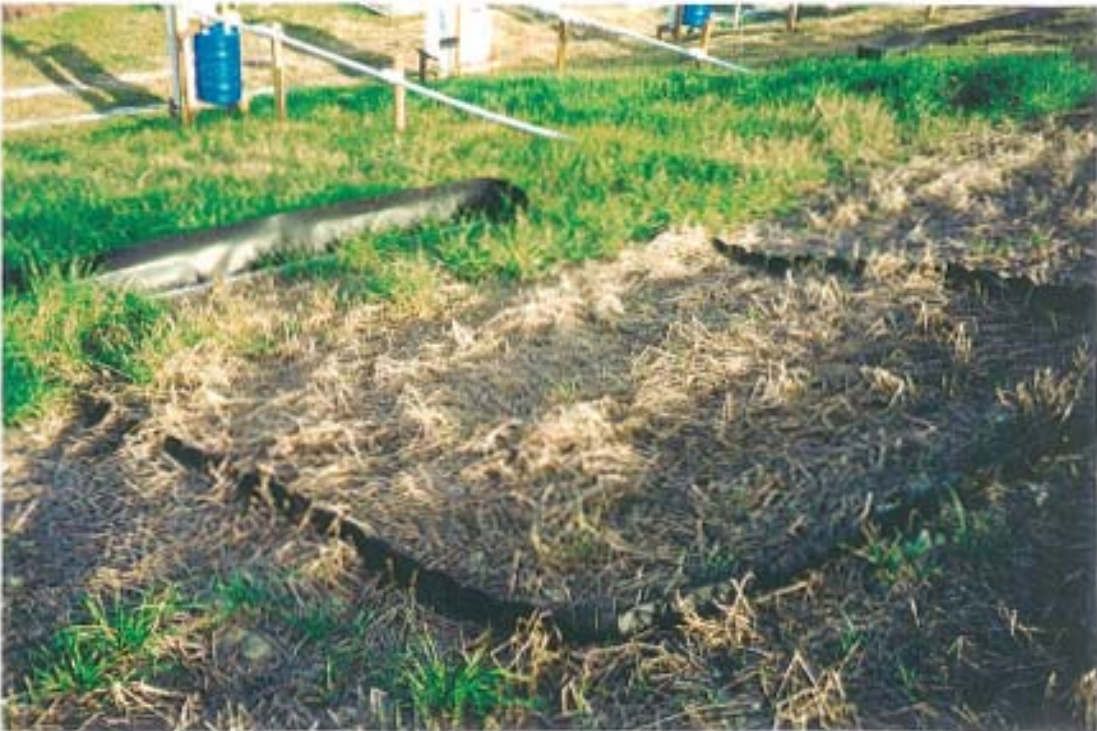
Photograph I-8. Side Slope Test Plot S2B on 01/13/99 (T=104 Days).
