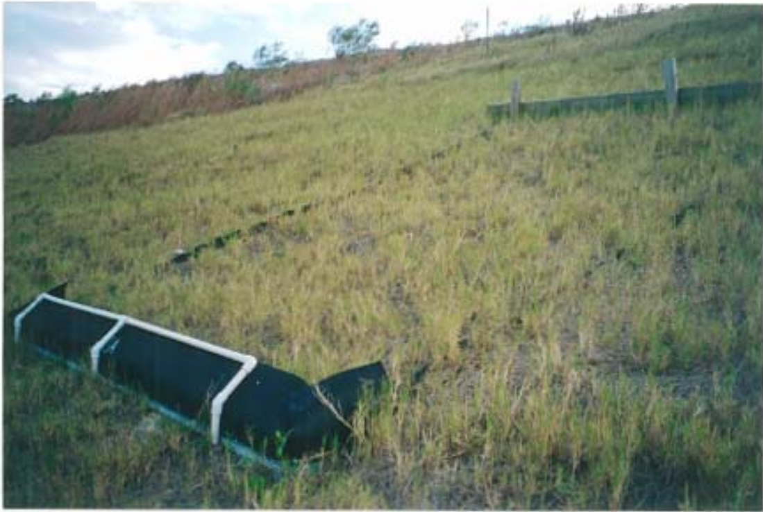
Photograph I-51. Side Slope Test Plot S1A on 11/14/01 (T=1140 Days).
