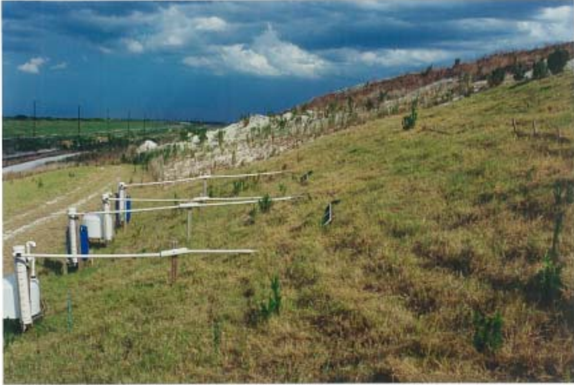
Photograph I-35. Side Slope Test Plot S1A on 06/19/00 (T=627 Days).
