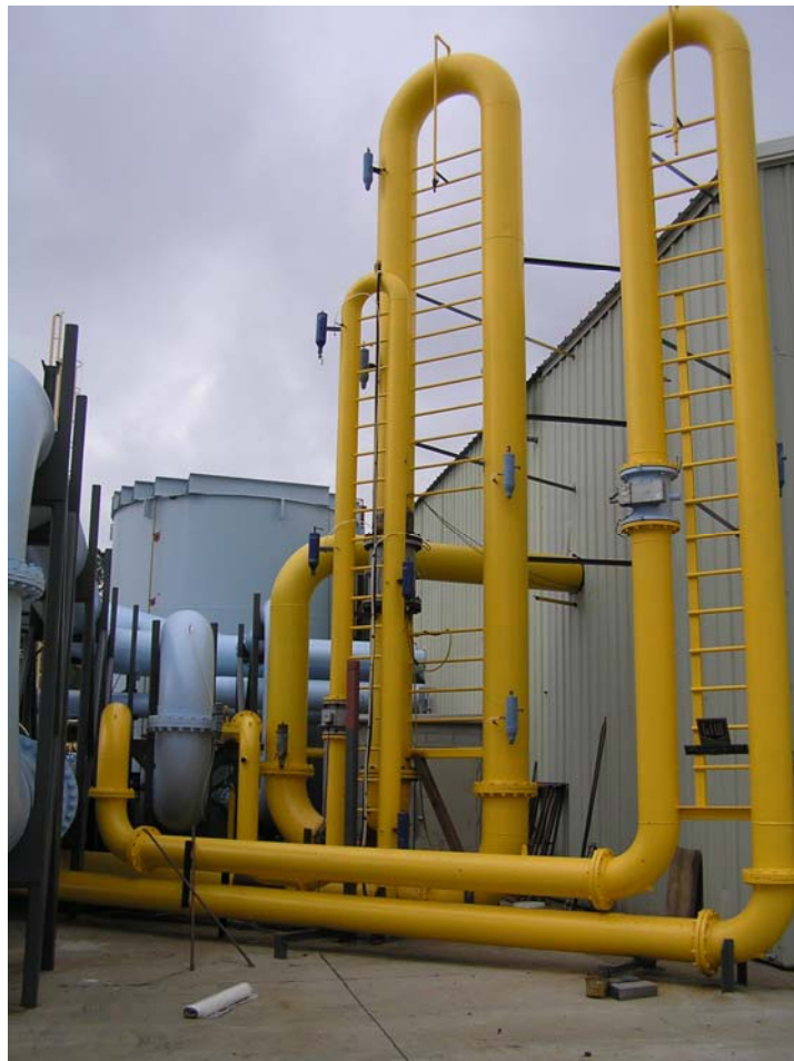
Figure D-5. Bend Flowmeter and SG Loop.
