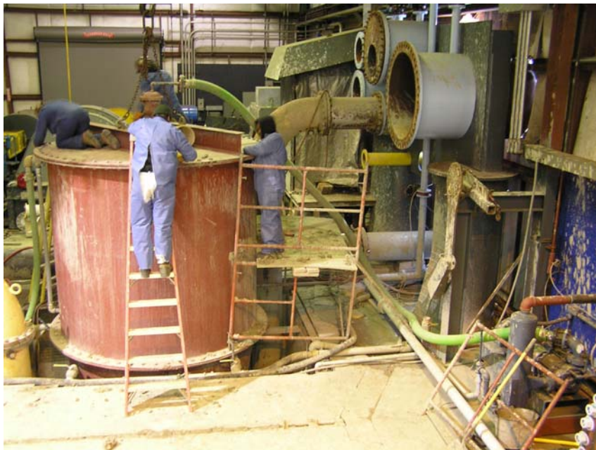
Figure D-7. Vacuum Pump and Sealable Slurry Tank.
