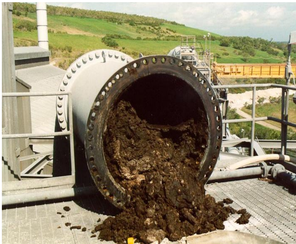
Figure 10. Pipe Removed to Clean Out Sludge
