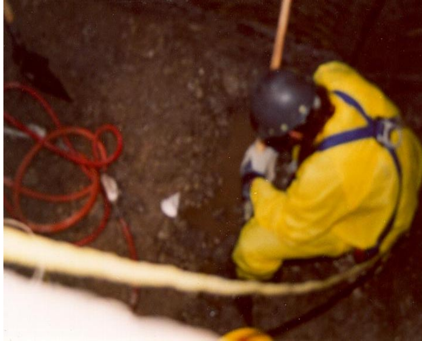
Figure 63. Reactor Cleaning: Hydroblasting
