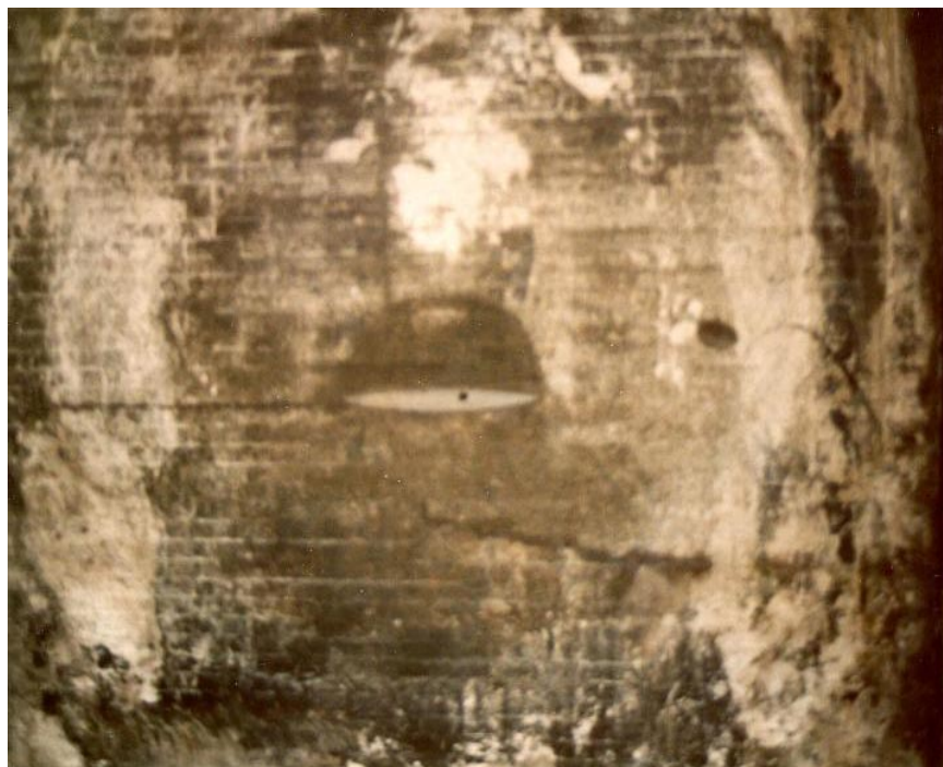
Figure 64. Reactor Cleaning: Cleaned Brick Lining
