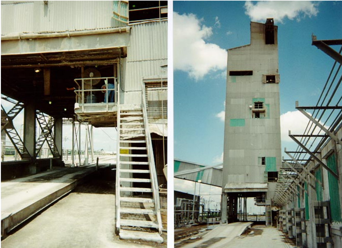
Figure 62. Truck Loading Station: Air Particulate Sampling
