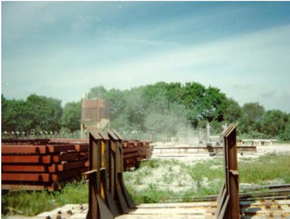
Figure 41. Paint Yard Storage - Open Environment
