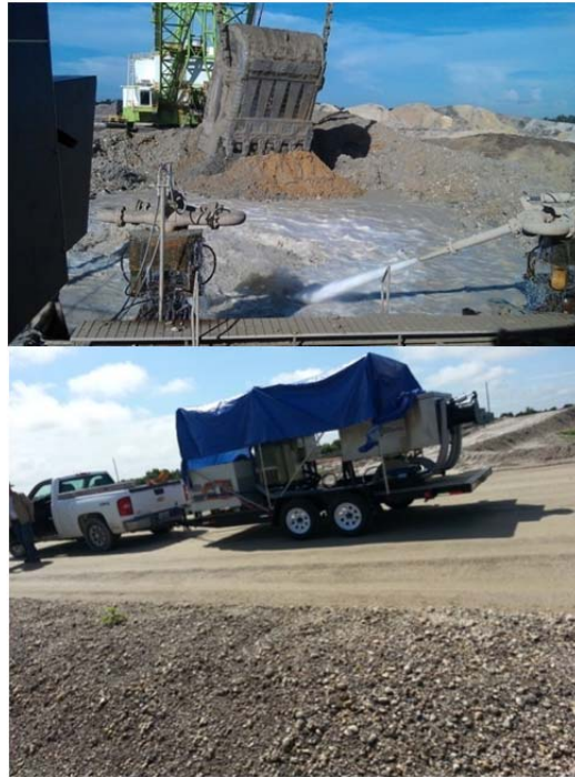
Figure 37. ReLIBS Unit Situated at Washing Pit Site Facing Matrix Rock Delivered by the Dragline.
