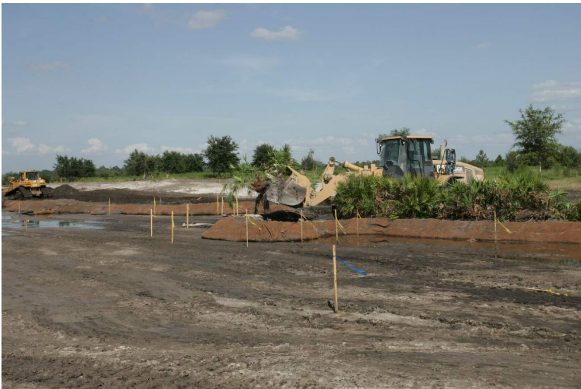
B) Built right bank above sub-grade and transplanting palmettos along bank.
