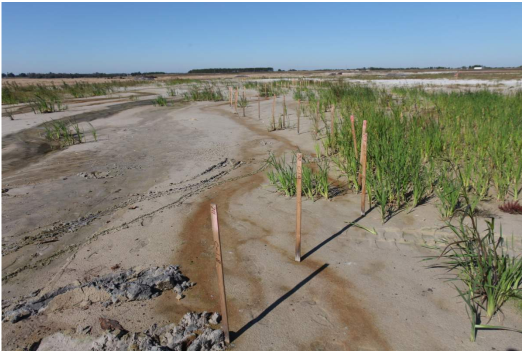
A) Floodplain contoured and stream channel alignment staked.
