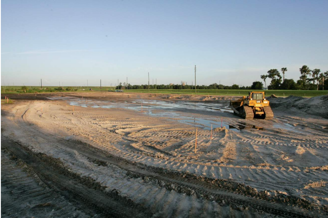
A) Filled-in existing canal and sub-grading the meander belt.
