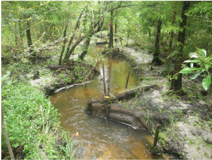
B) Wing deflector more than one month after installation.
