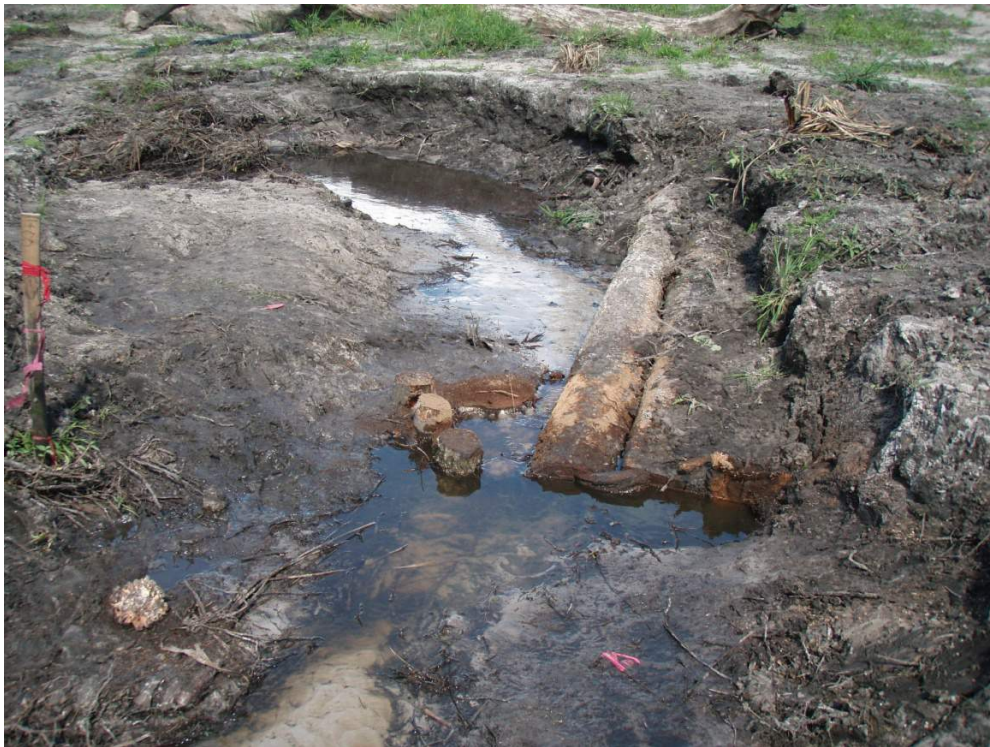
A) J-hook placed after 4 weeks of hydraulic carving to preserve bend.
