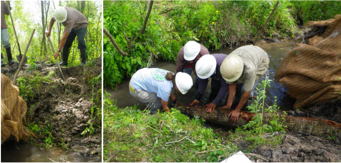
A) Manual labor installing wing deflectors and other LWD habitat amendments.
