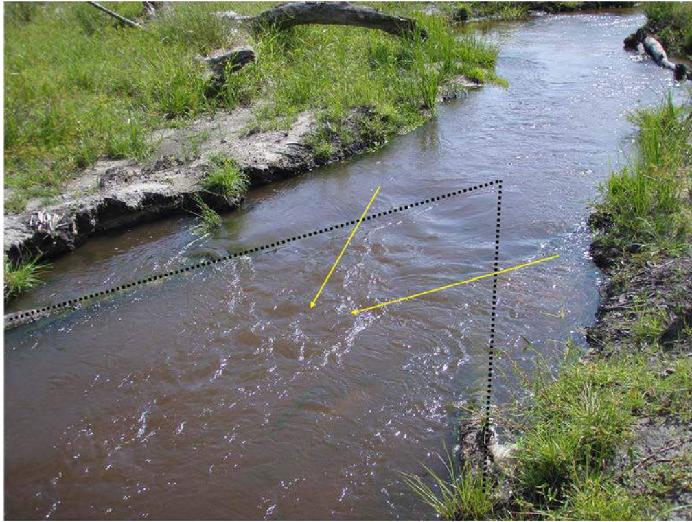
D) Same V-log weir submerged by bankfull discharge at equilibrium dimension. Dashed line shows location of logs and yellow arrows depict flow direction. DB-2, South Pasture Mine
