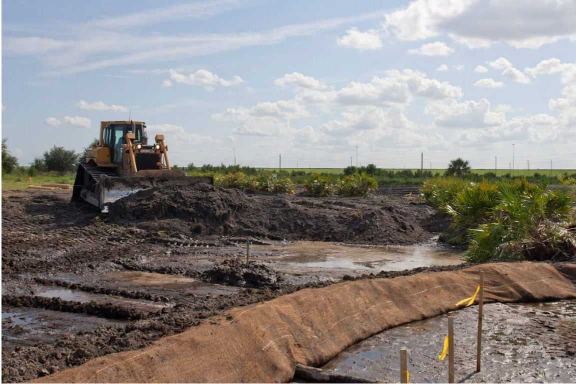
C) Placing meander belt soils in floodplain adjacent to bank.
