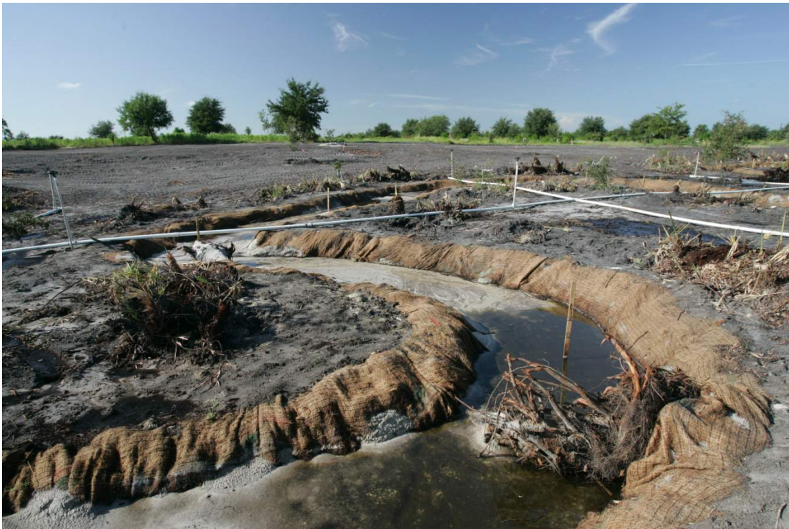
D) Both banks completed and all meander belt materials placed.
