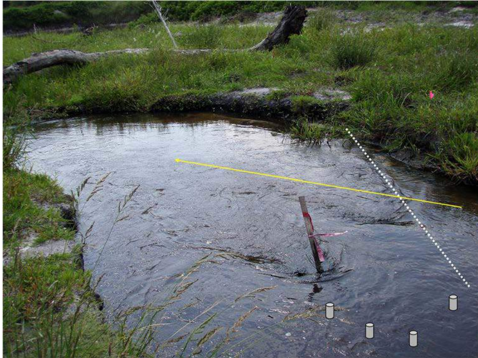
B) Same J-hook submerged by bankfull discharge at equilibrium dimension. Dashed line shows location of logs and cylinders show location of wood piles driven into the bed. Yellow arrow is flow direction. Note common survey stake with image A).
