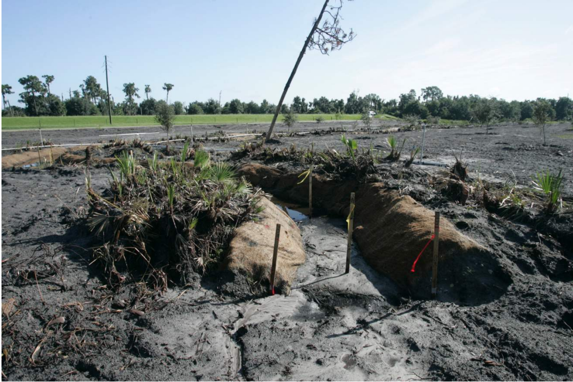
A) Head of channel immediately after construction with palmettos trimmed back.
