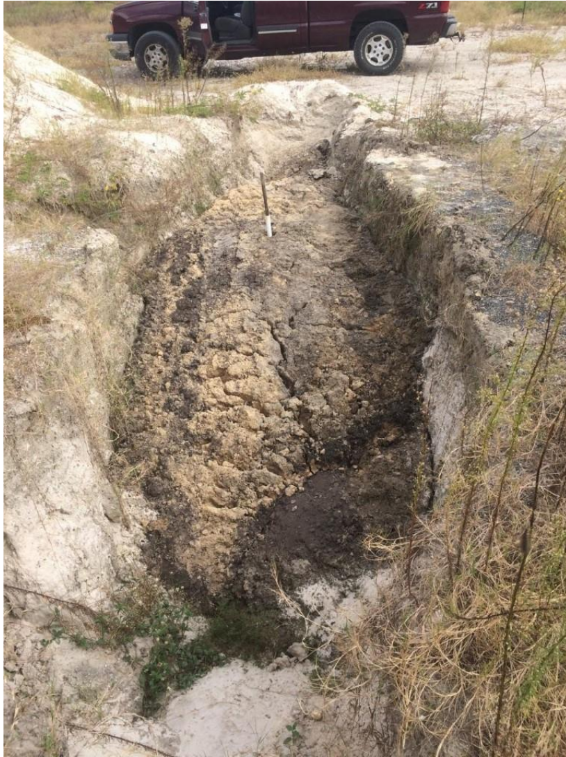
Figure 17: O:S:C Mix Placed in a Shallow Trench
