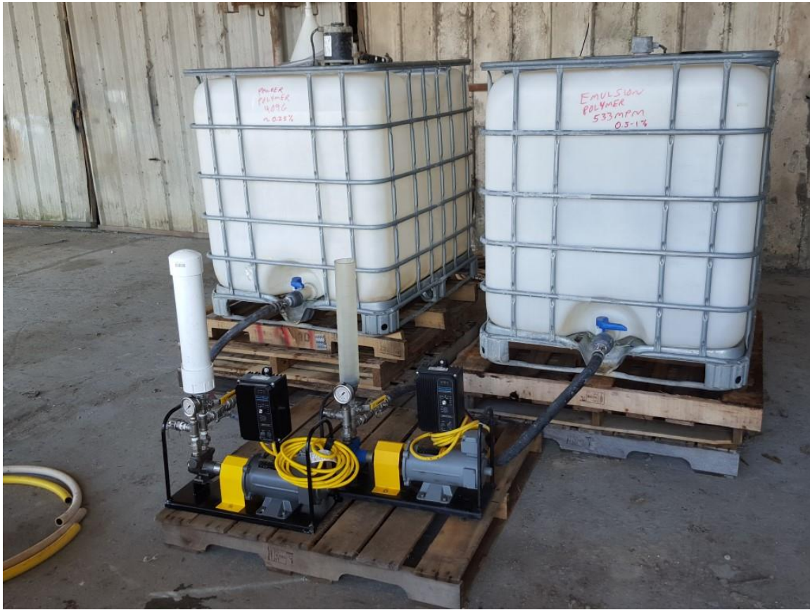
Figure 3. Reagent Tanks and Pumps
